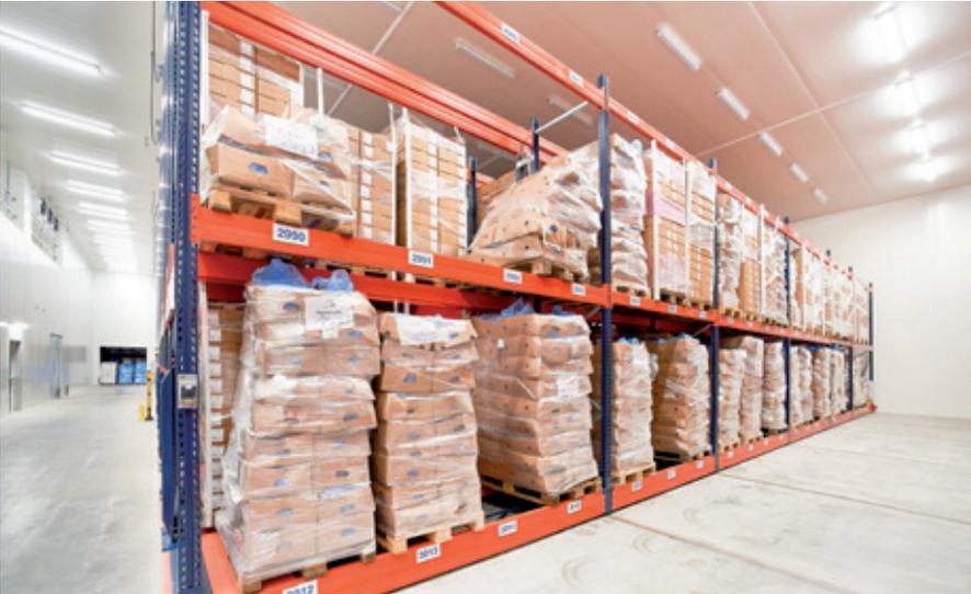
Comag has set up its frozen storage installation located in Mondovi (Italy) with two blocks of Movirack mobile pallet racking. This system ensures a storage capacity to house more than 2,000 pallets, without losing direct access to the merchandise.
