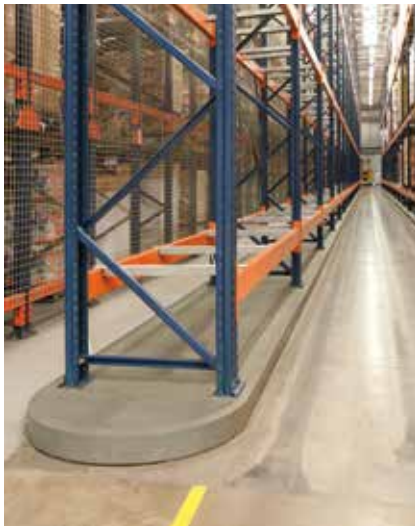
At the entrance of aisles with mechanical guidance, entry profiles with reinforced openings are installed to help centre the vehicles.
