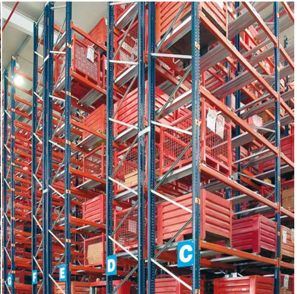
Selective pallet racking system with metal containers
