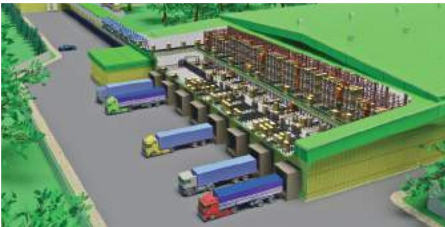
Aiming to keep pace with its growing business, the company Zbyszko wanted to expand the capacity and agility of their warehouse in addition to integrating their production and storage processes. In order to meet this demand, Mecalux built them an automated warehouse connected to the production plant via a 100 m long overpass equipped with conveyors. All this is coordinated and controlled by the warehouse management system Mecalux Easy WMS software.
