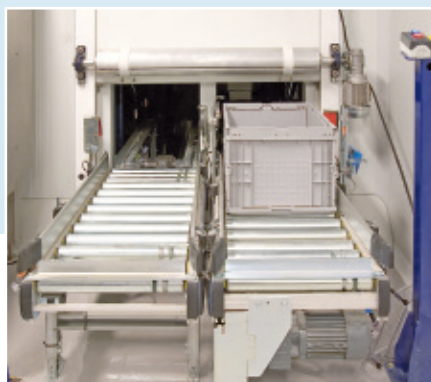
Automated Warehouse for Boxes
